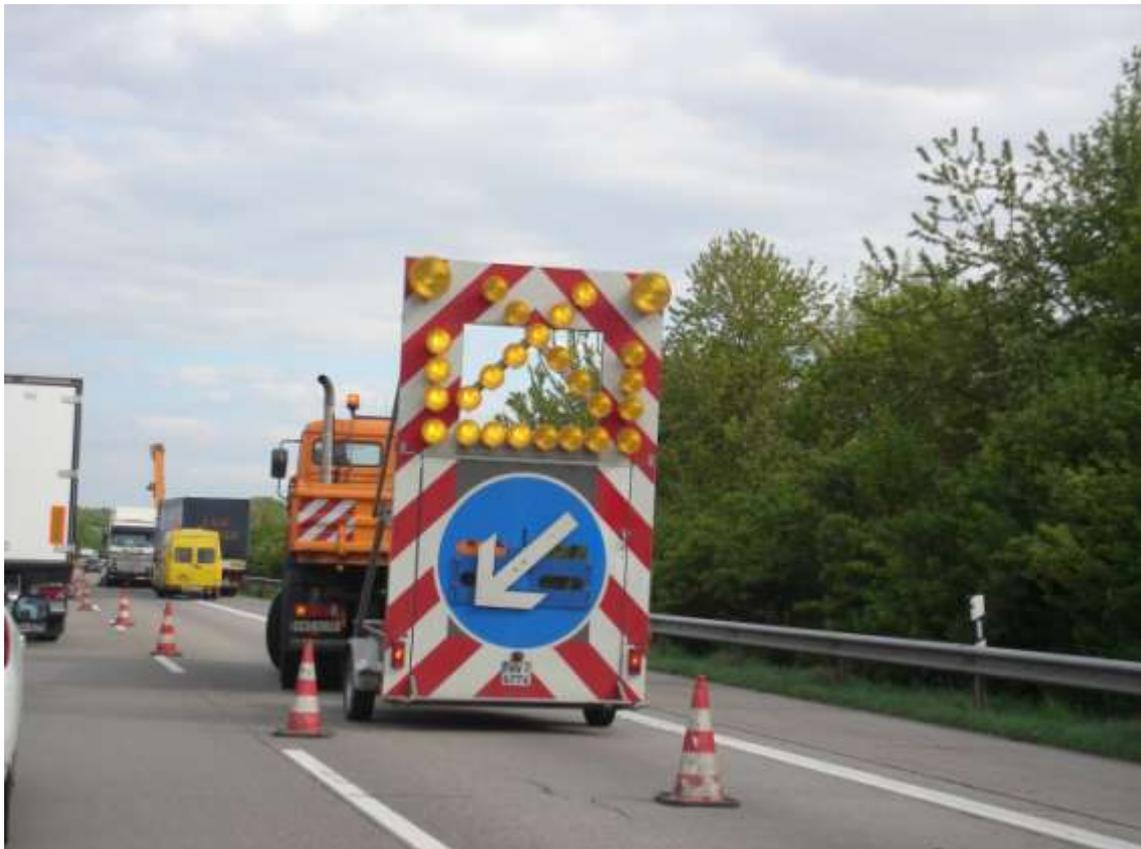
REMOLQUE CON FLECHA LUMINOSA EN CORTE DE CARRIL
